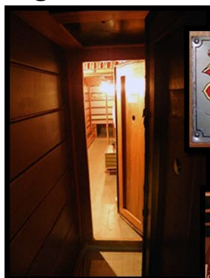
Double door air lock entrance to Universal Air Chest System
